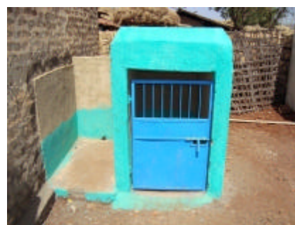
An Anganwadi toilet (not used)
