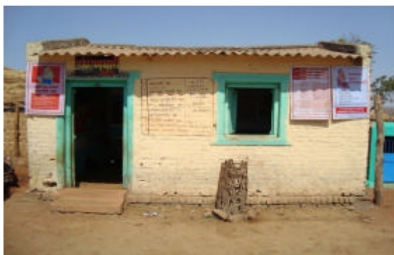
An Anganwadi structure -1
